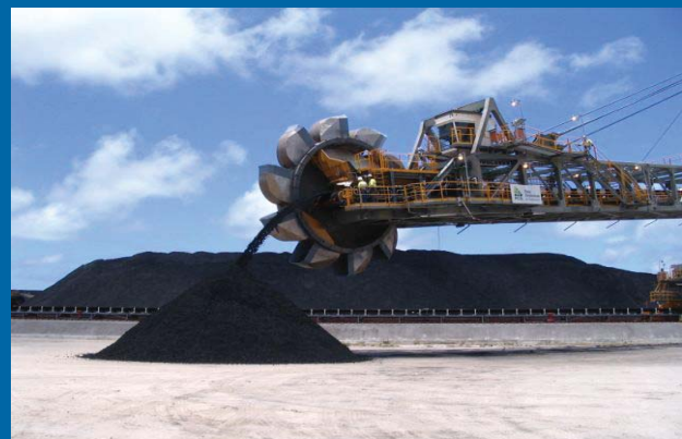
▲ Picture of trial running on site
