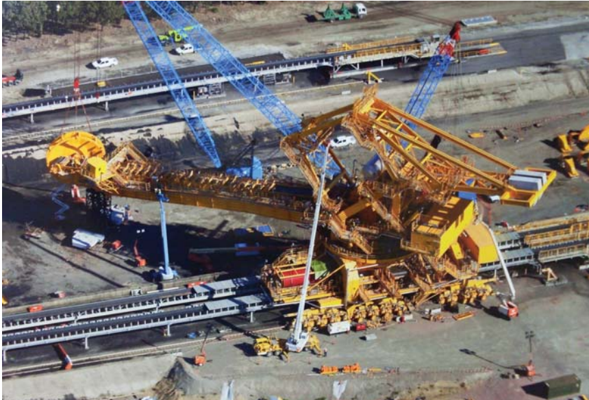
▲ Picture of trial running on site
