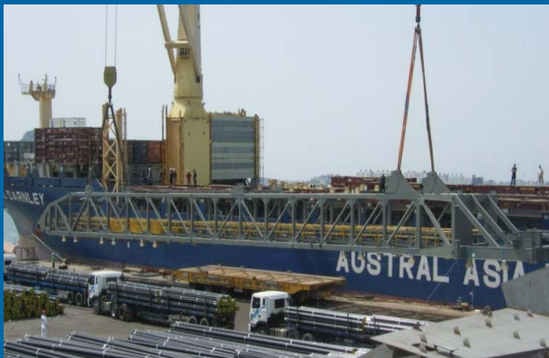
▲ Ship loading : B/W BOOM (Weight : About 120ton)
