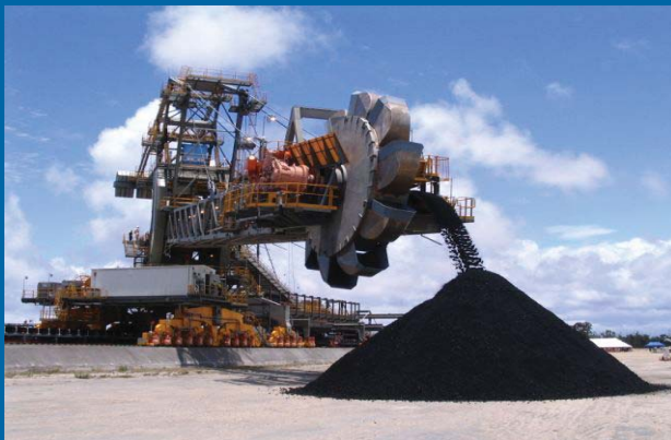
▲ Picture of trial running on site
